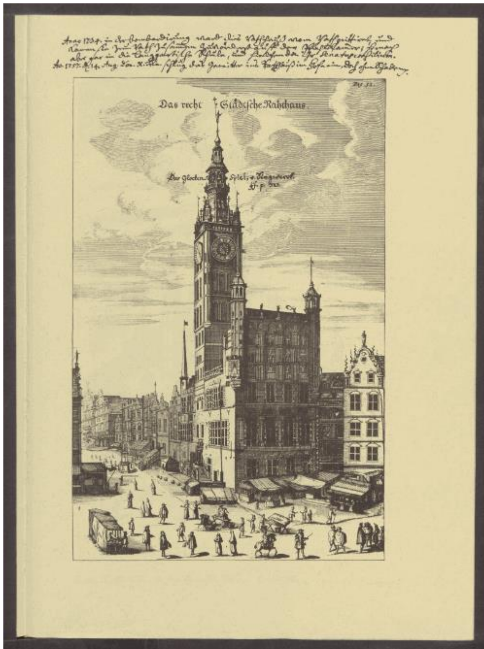
the Main City Town Hall in Gdańsk. Curicke, Der Stadt Danzig, 52.
